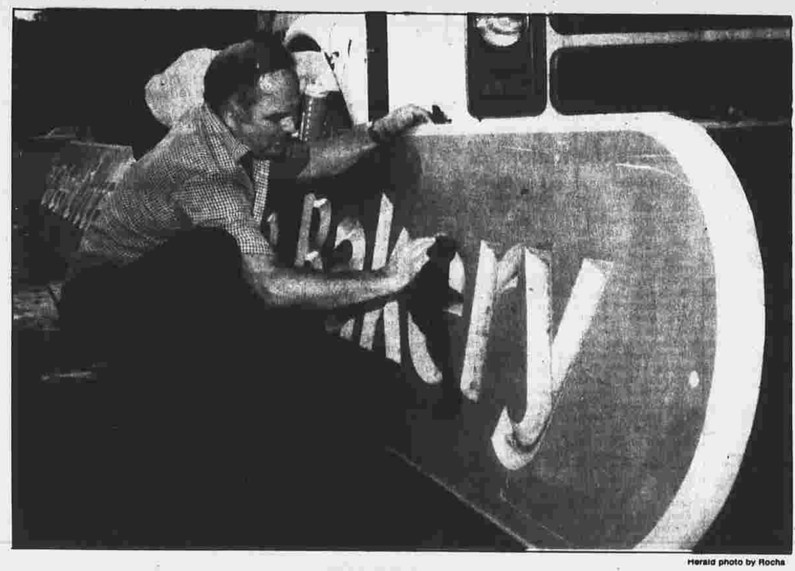
Maurice Bolduc of New Britain cleans new fiberglass signs at the Super Stop & Shop supermarket on Broad Street. He and a co-worker from the Saxton Corp. removed the old signs before hanging the new on Tuesday.
